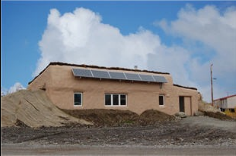
Anaktuvuk Pass prototype: Super insulated home with thermal-raft foundation
