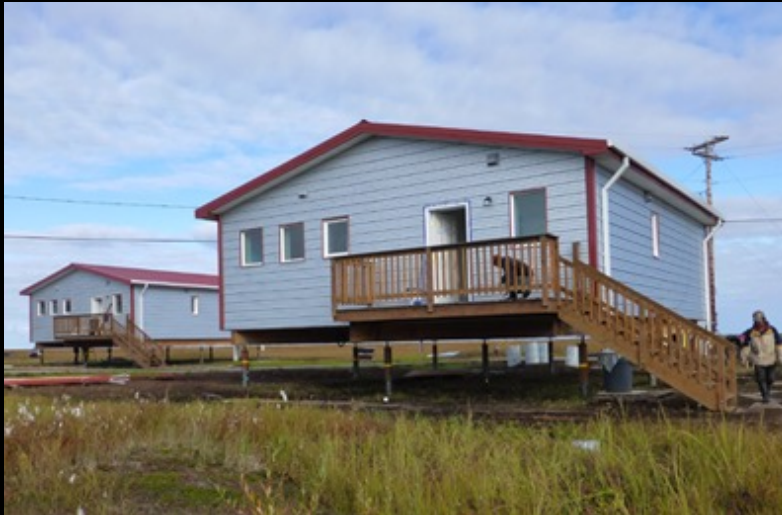
Atmautluak prototype: Integrated truss house, adjustable piling foundation
