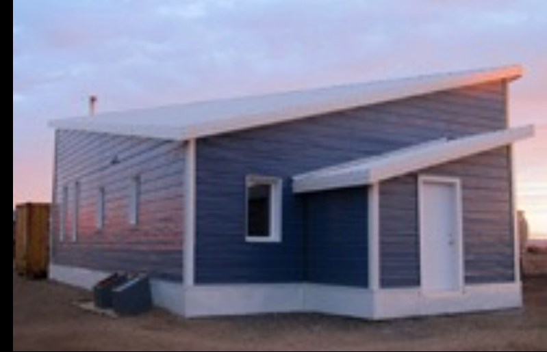
Buckland prototype: Thermal raft foundation, integrated truss house with single-piece, floor, walls, roof adjustable piling foundation
