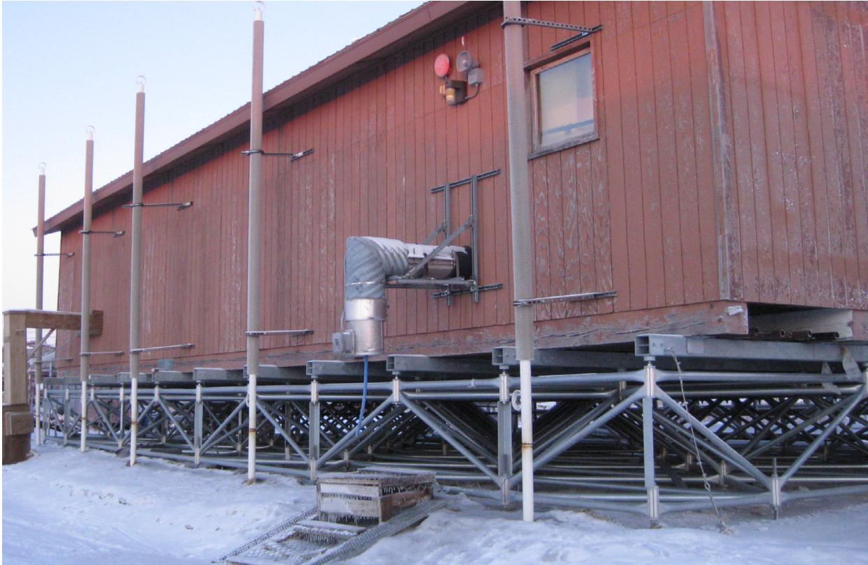
**Figure 21. Space frame foundation with thermosiphons in Atmautluak.
