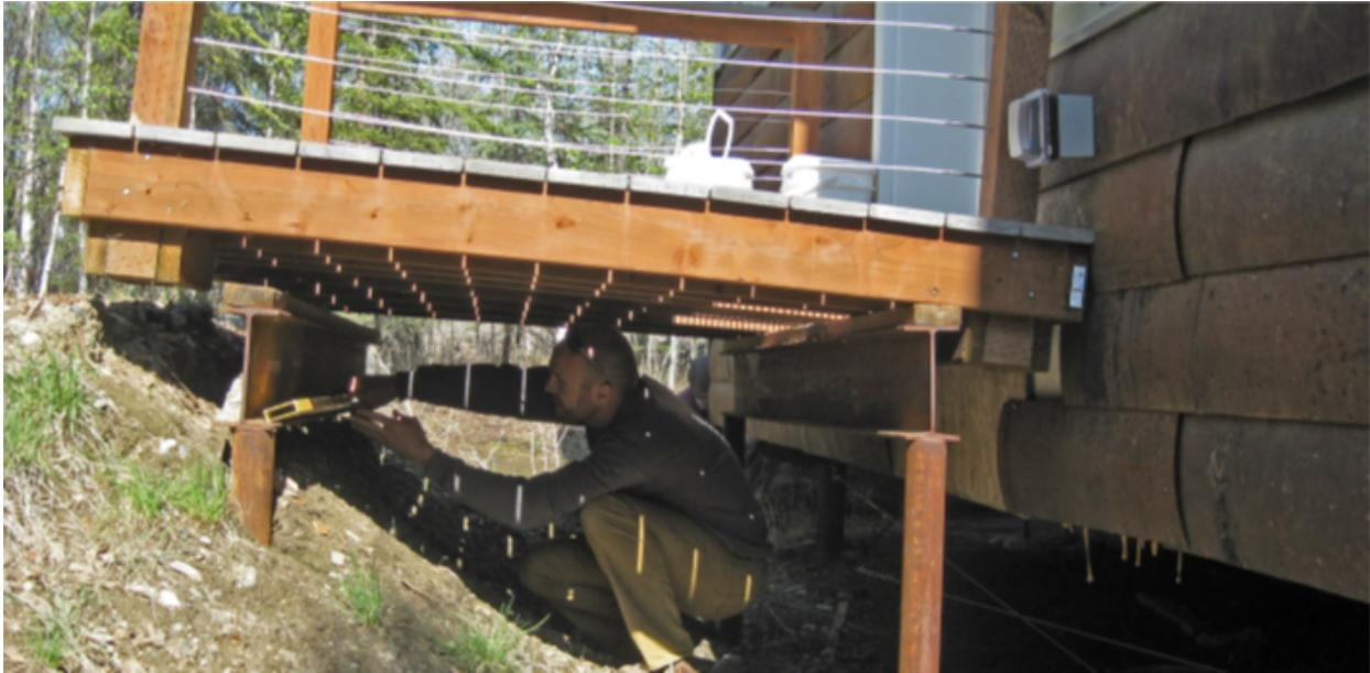
**Figure 3: Example of frost jacking. (CCHRC Inc.)**
