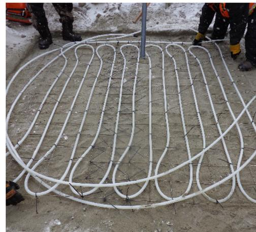
**Figure 23. Active cooling loops laid under a slab on grade commercial foundation. (CCHRC Inc.)**
