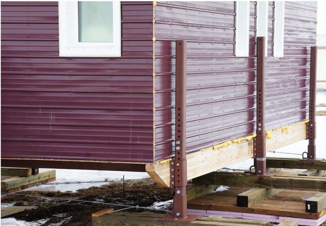
**Figure 26. Adjustable foundation example. (B. Tracey, Point Lay)**
