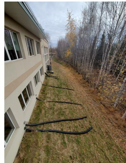
**Figure 24: (left) Gutters and a downspout help direct rain and snow-melt. (right) Drain spouts and flexible drain channels direct water away from the building and into a ditch that feeds a retention pond (in the distance). (G. Davis, NREL)**
