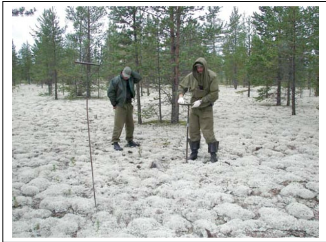
Figure 12. Installation of the temperature sensors and mini loggers at the ND PiCla site.
